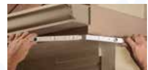
Fit Magnet Tracks together, change magnets spacing on back.
